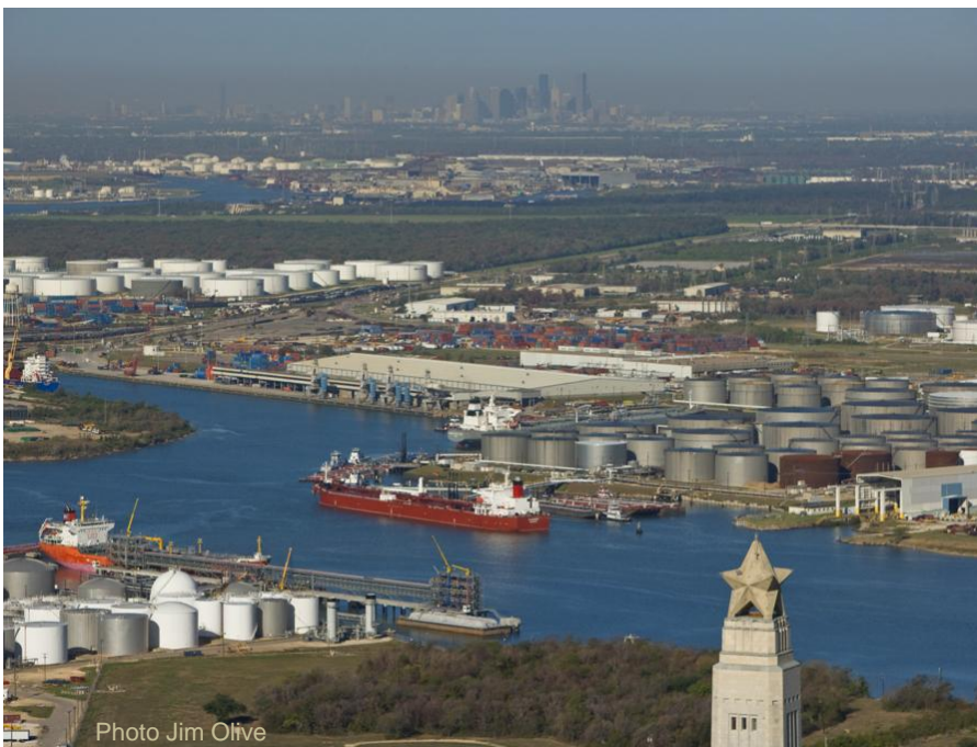
Low-lying tank farms adjacent to the Houston Ship Channel. Photo by Jim Olive.
